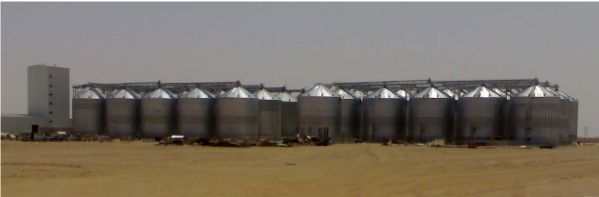
90,000 tonne Maize Silos – expanded from first phase of 30,000 tonne with Feed Plant (Saudi Arabia)
