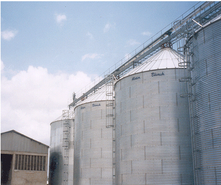
10,000 tonne Wheat Silo Plant (Tanzania)
