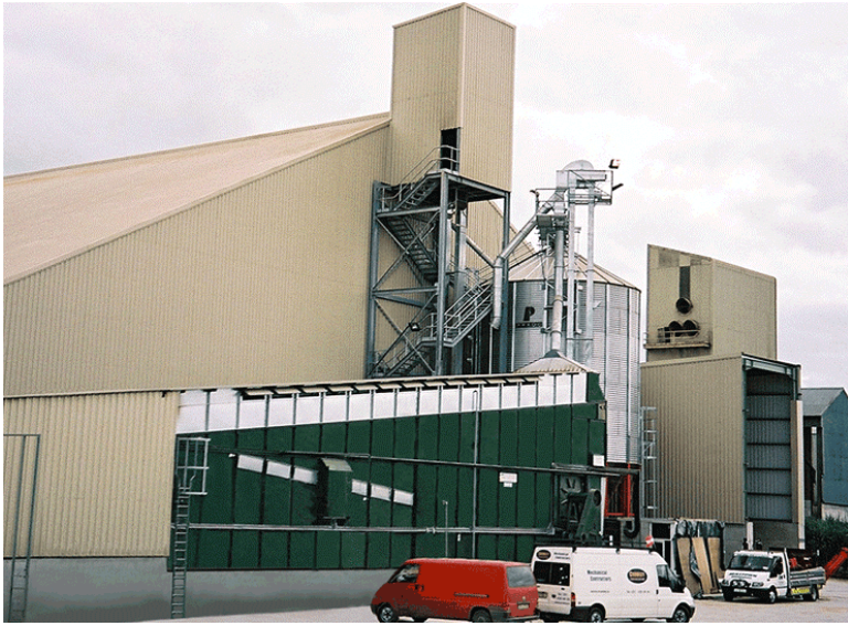
Double Flow Drier 70t/hr- with pre- drying silo (Ireland)
