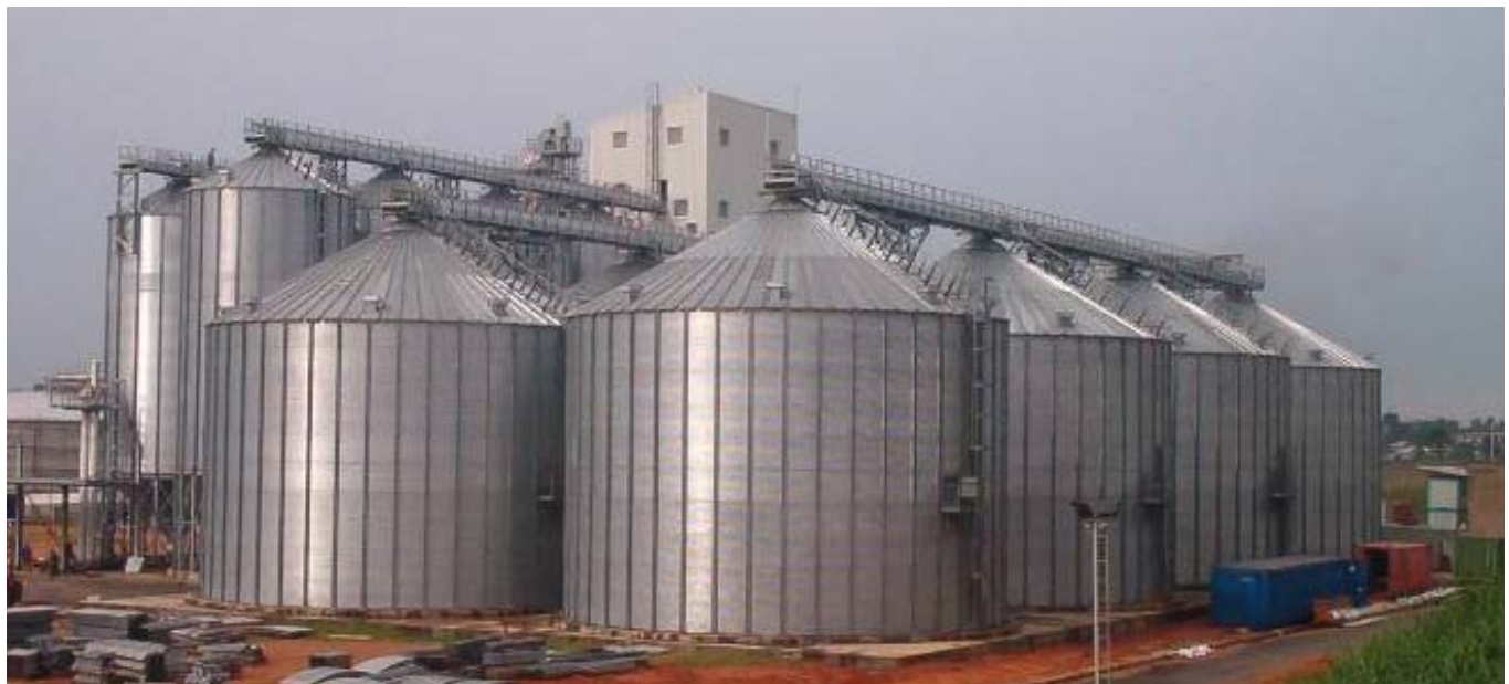
10,000 tonne Symaga silos installed by Alvan Blanch Nigeria (Aba)
