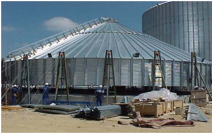
12,000 tonne Symaga silos installed by Alvan Blanch Nigeria (Libya)
