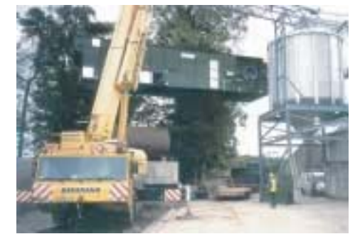
Main section of SPD 42000 Drier - lifted from truck to final position
