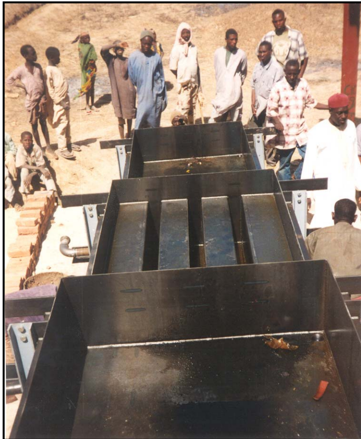
Assembly of the four-stage boiling vessel system
