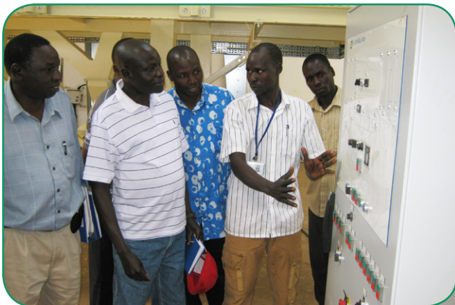
Discussion of control panel during handover
