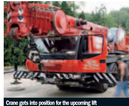
Crane gets into position for the upcoming lift
