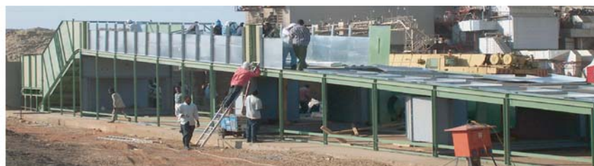
(SFD 18/12) Drier under construction in Sudan
